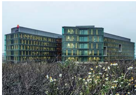
Head office PriceWaterhouseCoopers, Gasperich, Luxemburg BREEAM Very Good / Completion 2014 ETAP solution with UT1 recessed luminaires, R8 and R4 mounted luminaires and E6 industrial luminaires.
