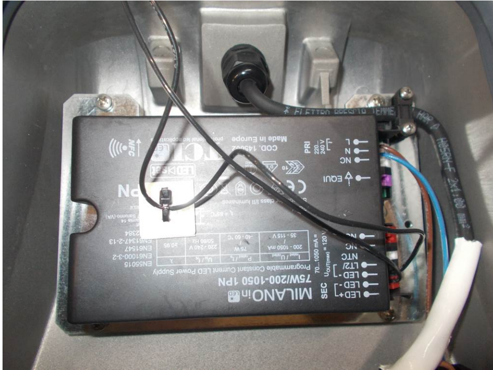
Pic.10: internal view
