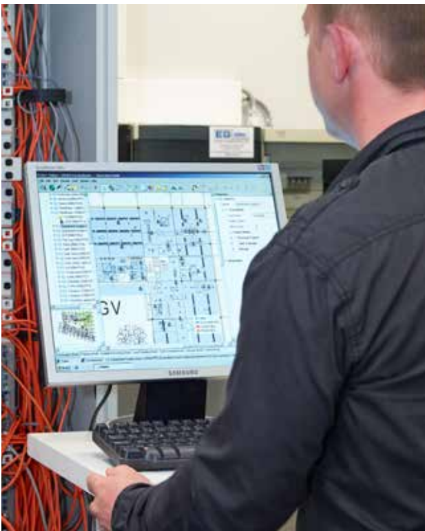
Commissioning of the light management system.
